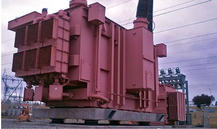
Figure 11: Transformer retrofitted with base isolation [4]
